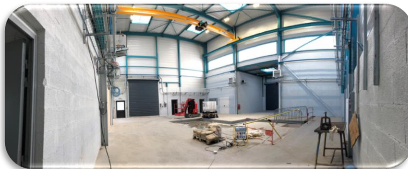
SIDERWIN pilot plant building
