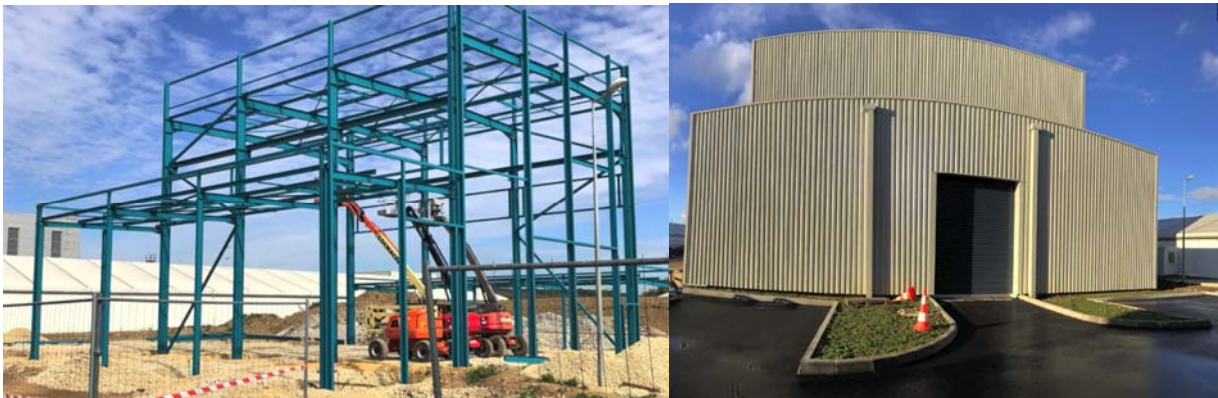
Figure 15. Pilot Plant Building construction
