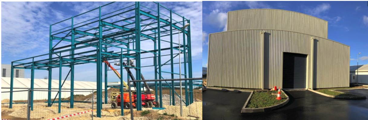
Figure 21. ΣIDERWIN Pilot Plant Building erection
