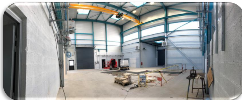
SIDERWIN pilot plant building
